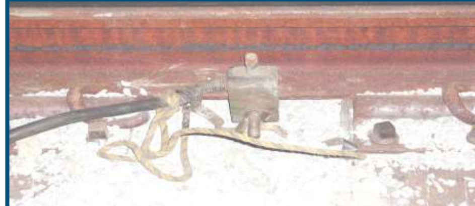
Ground stick cable attached to rail
