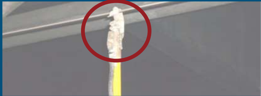
Ground stick hung on catenary (trolley) wire, residual power runs down cable into rail.
